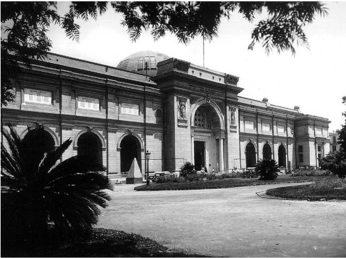
41 - Le musée des Antiquités, place Ismailya architecte Marcel Dourgon (1902) 41 - Antiquities Museum, Ismailya Square architect Marcel Dourgon (1902)
