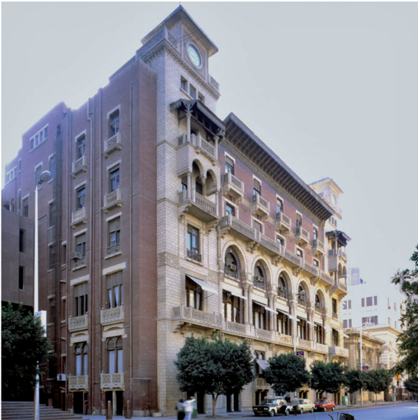
122 - La banque Misr, 151, rue Mohammad Farid, architecte Antonio Lasciac (1927) 122 - Bank Misr, 151 Mohammad Farid Street, architect Antonio Lasciac (1927)
