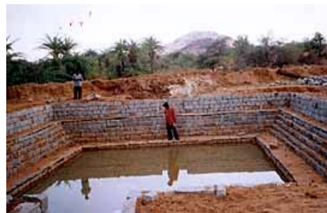
Tank at Kothagudikunta
