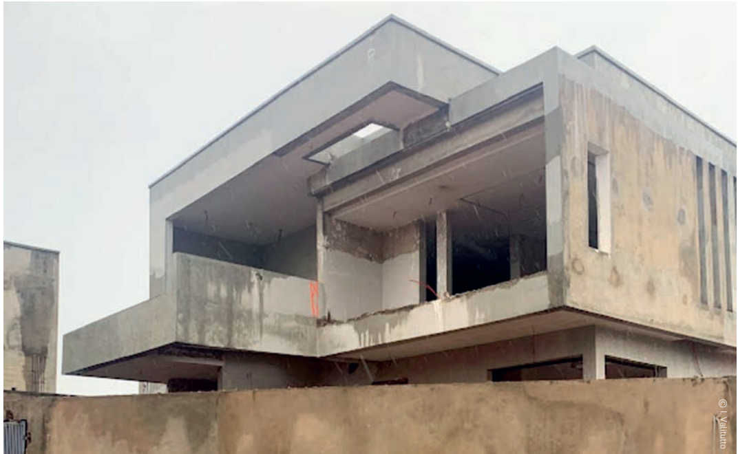
Construction in progress on the Renaissance residence (Lomé, October 2023).
