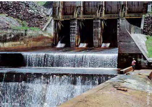
Rio Pitinga dam, Brazil.
